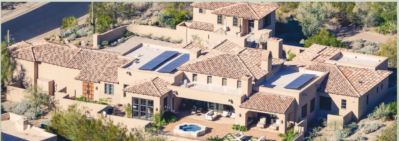
A triple-string concealed rooftop solar electric array adorns this LEED certified custom luxury residence located in North Scottsdale.
