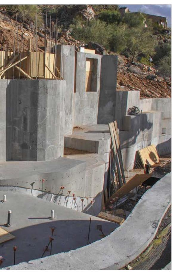
**LEFT:** Concrete reinforced support walls hold back the mountain. According to Meek, the concrete used on this project has a compression strength of 7,000 pounds per square inch. In comparison, the typical footing on a house can be as low as 2,500 psi, he notes. The pool's walls are also designed to withstand the Valley's extreme temperatures
