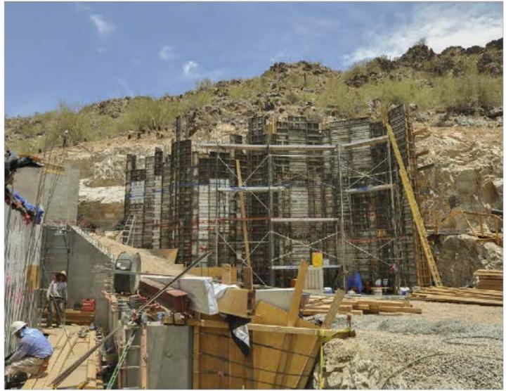
**ABOVE:** One hundred and sixty truckloads of concrete (1,500 cubic yards) were used to construct the structure, which included retaining walls as tall as 32 feet.
