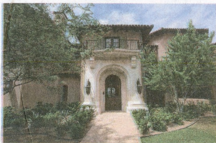
Other energy-efficiency features help to enhance the Silverleaf home's geothermal system.
